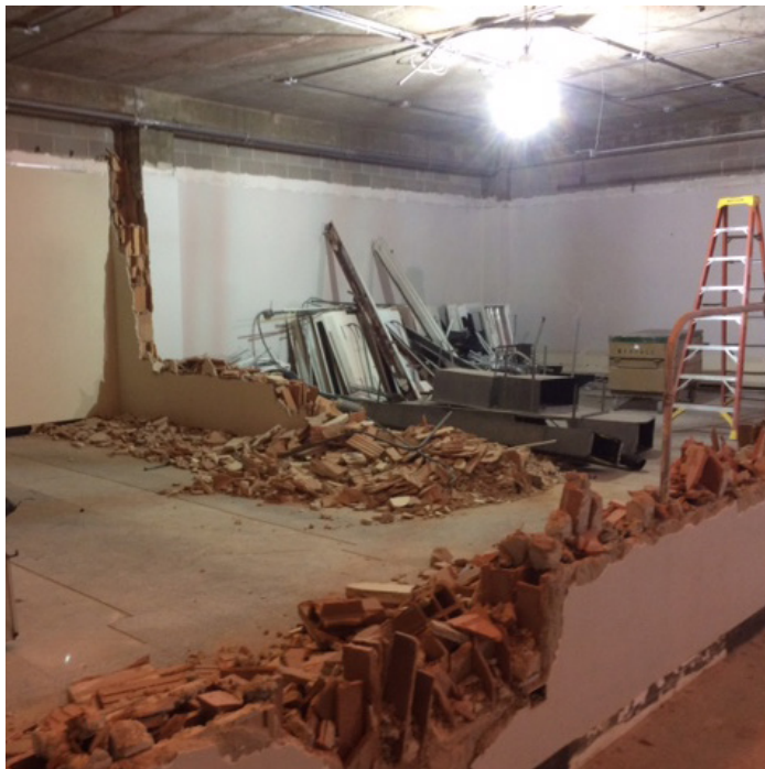
Demolition of the University Archives in progress
